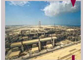
Gas treating & liquefaction
