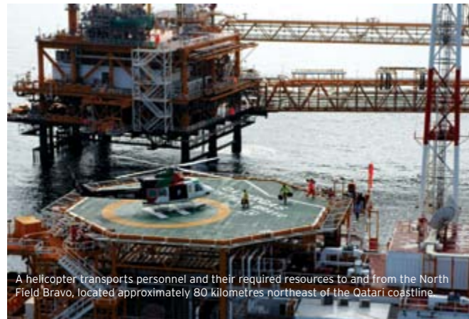
The Qatargas offshore facilities at North Field Bravo.
